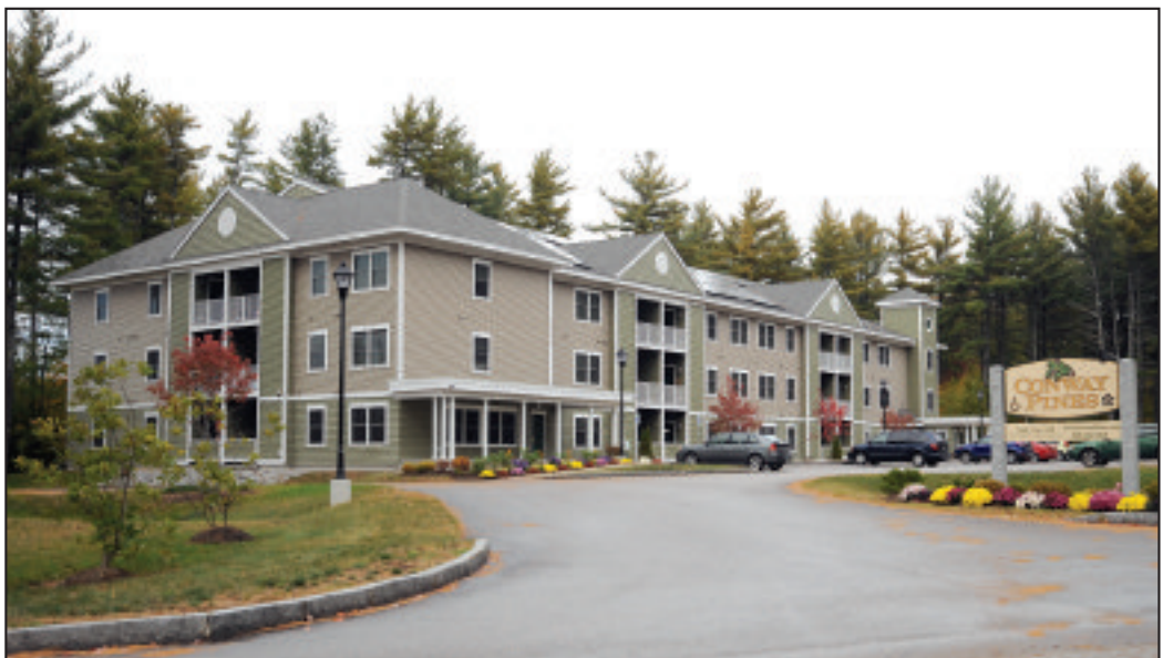
The senior housing building will go up next to the Conway Pines affordable workforce housing (above). (JAMIE GEMMITI PHOTO)
